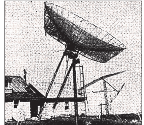
Moonbounce antenna – the 27-foot diameter parabolic dish built by Mr. Vic Michael, W3SDZ , of Williamsport, Pa.; a measure of the initiative and dedication of moonbouncers.
